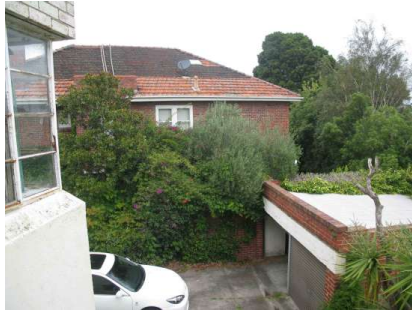
(J) GARAGE VIEW
