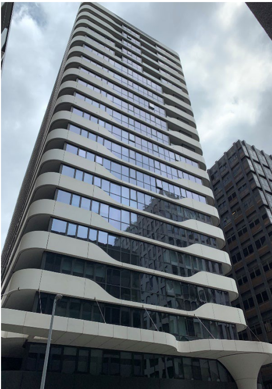
16. 12 Queens Road rear elevation to lane
