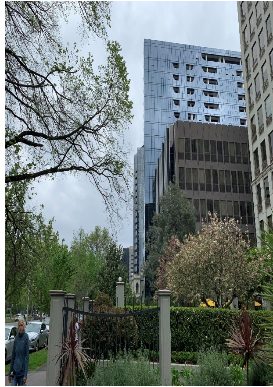
05. View from subject site frontage looking south
