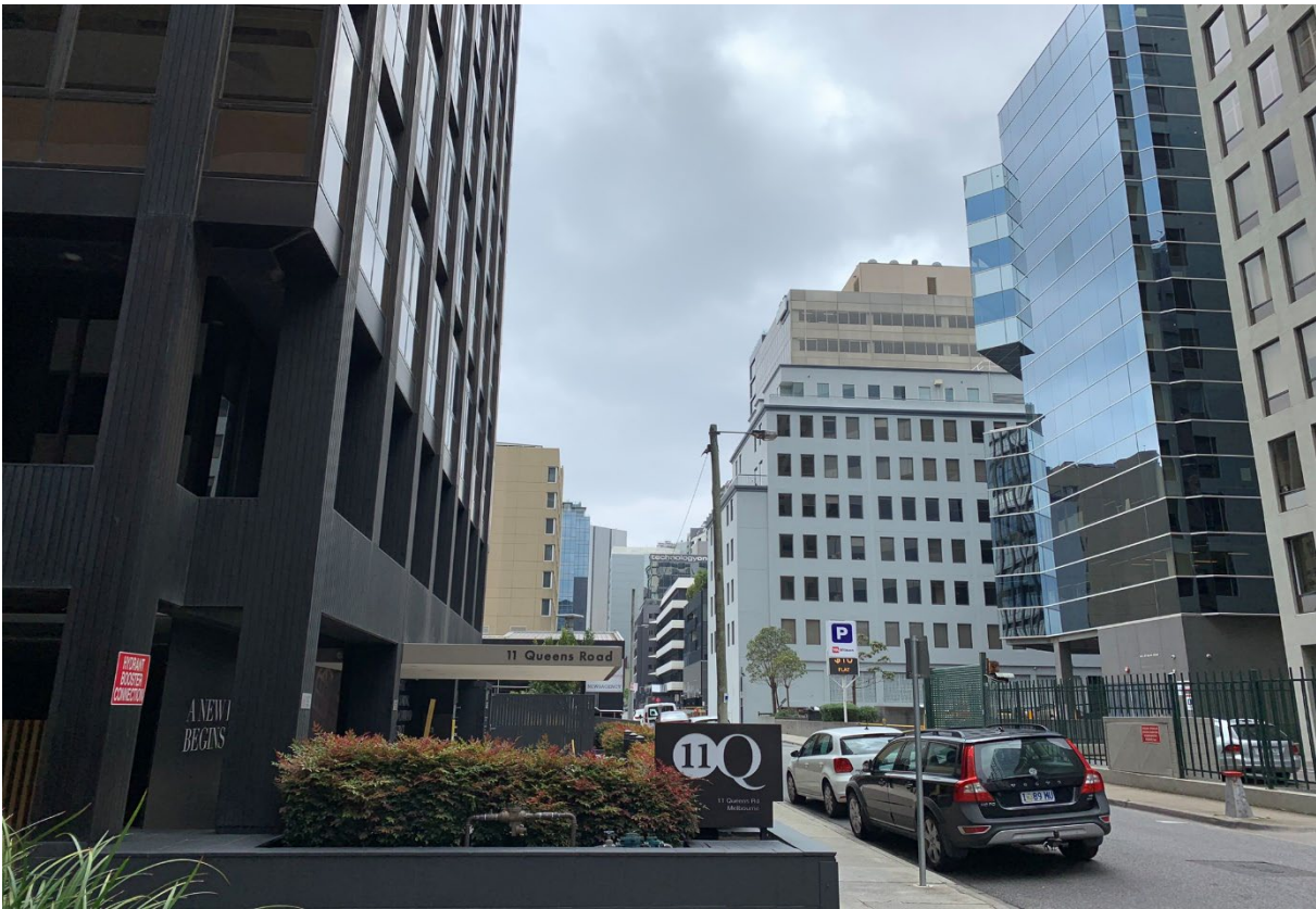
20. 11 Queens Road angle elevation to lane
