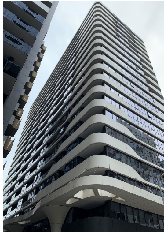
17. 12 Queens Road - Lane balcony view
