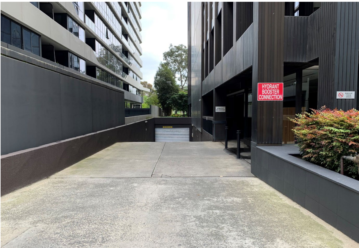
21. 11 Queens Road entrance to basement from lane
