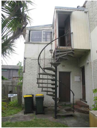
(F) REAR EXTERNAL SPIRAL STAIRCASE
