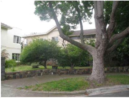
(B) 21 HOLROYD AVENUE STREET VIEW
